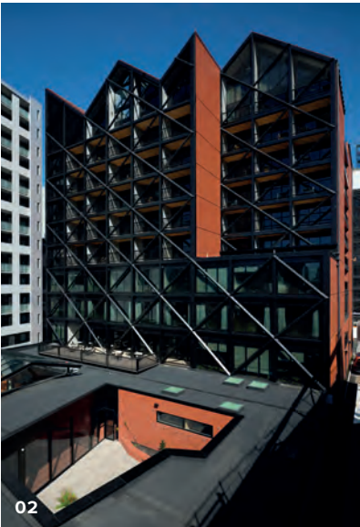
01 Most of the floors are mass timber panels braced laterally by the steel lattice that gives the building its distinctive frontage. 02 The east view from Federal Street includes the courtyard of Hobson Street’s ground level.
